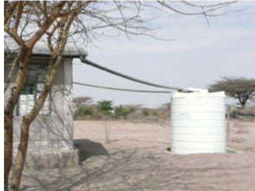
Fig1: Rainwater is collected from the roof
