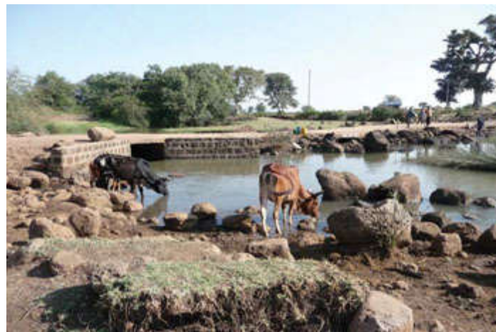
Fig2: Surface water source
